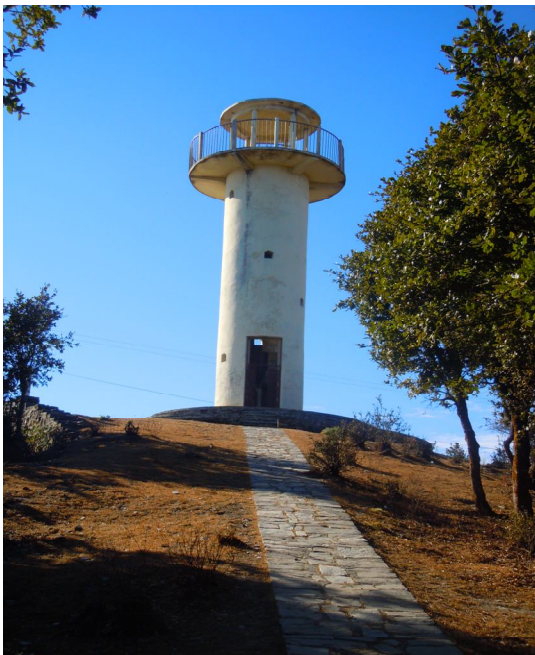
View tower at the top
